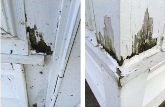
Location: Cottage window trim The trim is rotting. Repair or replacement is recommended.
