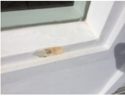
Location: Cottage window trim The trim is rotting. Repair or replacement is recommended.
