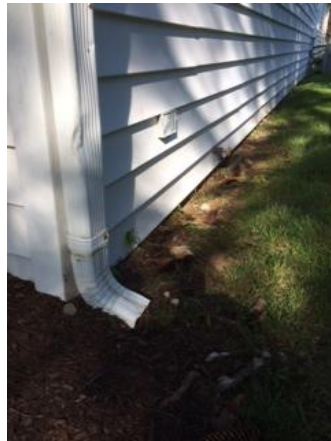
Locations include, but may not be limited to: NW inside corner of the house, cottage The negative grade should be corrected. Site drainage and roof runoff management should be optimized.
